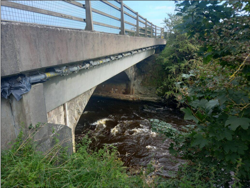
Plate 3-19 Water crossing 2 over the Clare River
