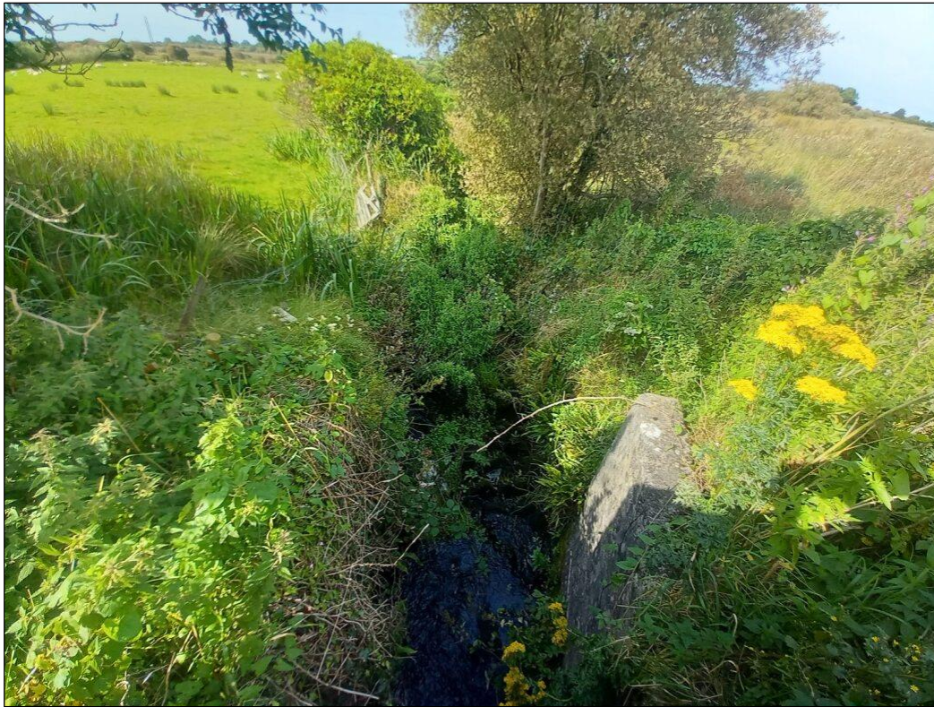
Plate 3-21 Water crossing 4 over Clare River tributary
